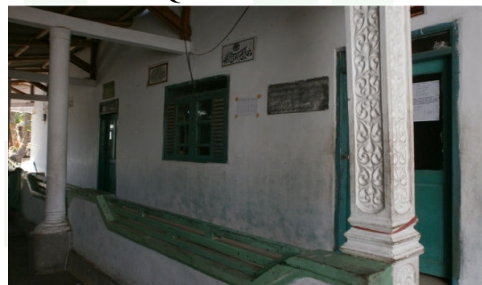
Bagian Samping TPQ Nurudz Dzolam
