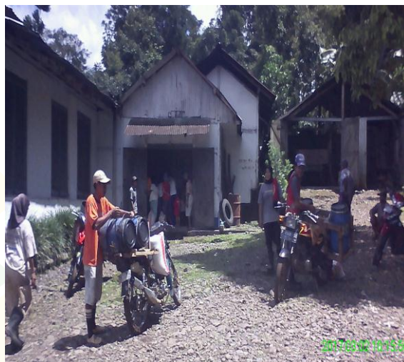
Koperasi PT. Kalianda Concern
