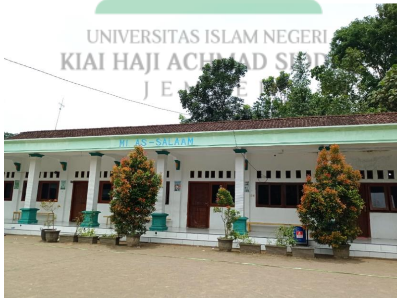
Gambar 4. 1 Gedung Madrasah MI As salaam
