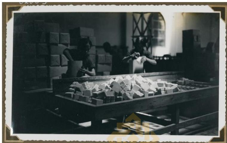
**Gambar 1.5** Pengemasan briket garam di Tordjeon, Sampang
