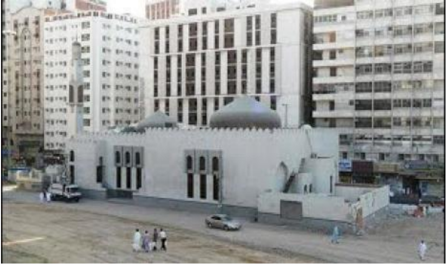
Gambar 20: Masjid Kucing (Ar-Royyan) di Makkah
